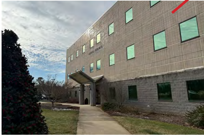
Facade improvements required
