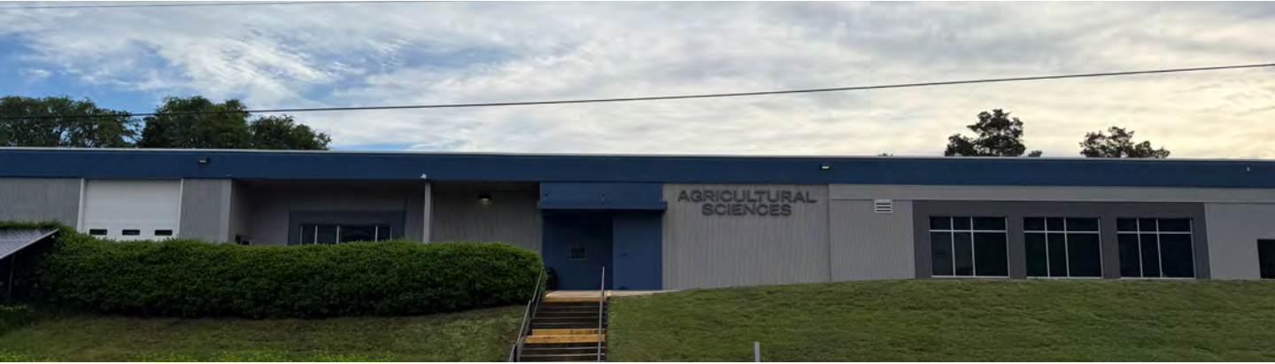
EXAMPLE OF SUCCESSFUL FACADE IMPROVEMENTS THAT WILL BE EMULATED
