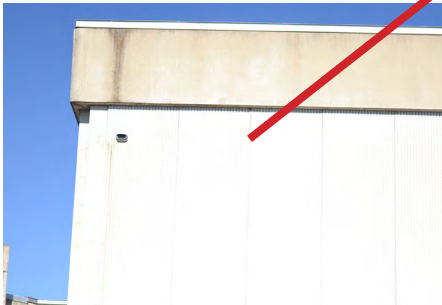
Application of exterior treatments
